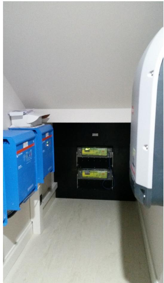
The medical centre also installed a 30 kW PV solar array. Due to the roof angles and space this was installed on an east - west array. The PV array is supported by 2 x Fronius inverters, one for the east array and one for the west array. The SoNick batteries are supported by 3 x Victron inverters with an inverter on each phase.
